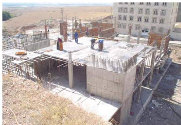
New Quality pilot project – construction site (BHRC)
